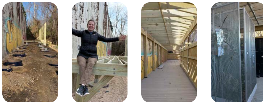
ABOVE: Progression of the outdoor deck build over the winter
